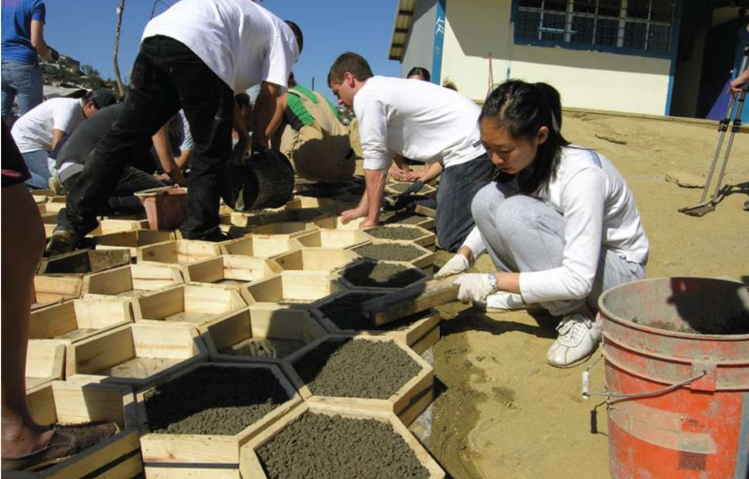
Students from UCSD Urban Studies and Planning Program's Student Club working on the pervious pavers on the elementary school playground of the Colonia San Bernardo, a low income neighborhood in the Los Laureles Canyon Project area.
