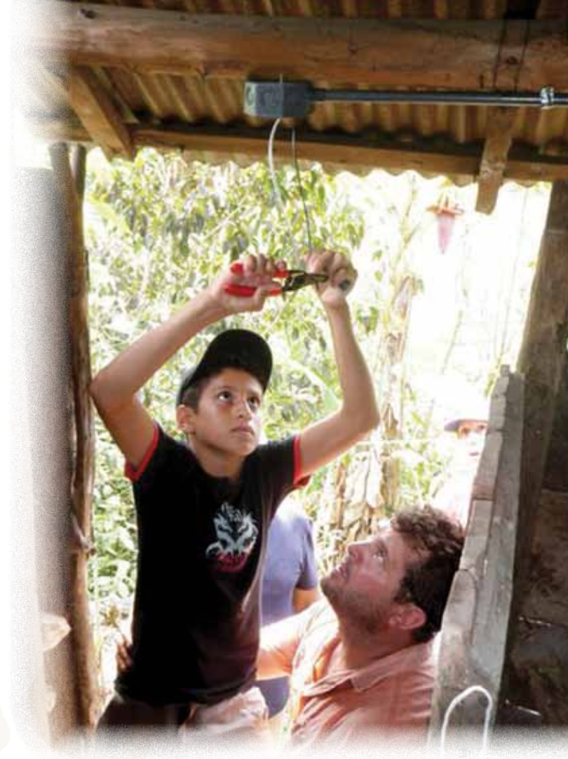
Madison College Renewable Energy for the Developing world program participant helps teach a local youth how to wire a light socket in a home that has never had electricity.
