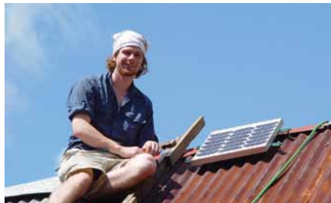
Madison College Renewable Energy for the Developing World participant checks the installation of a small PV panel that will provide lights for a family on the Zapatón Indigenous Reserve in rural Costa Rica.
