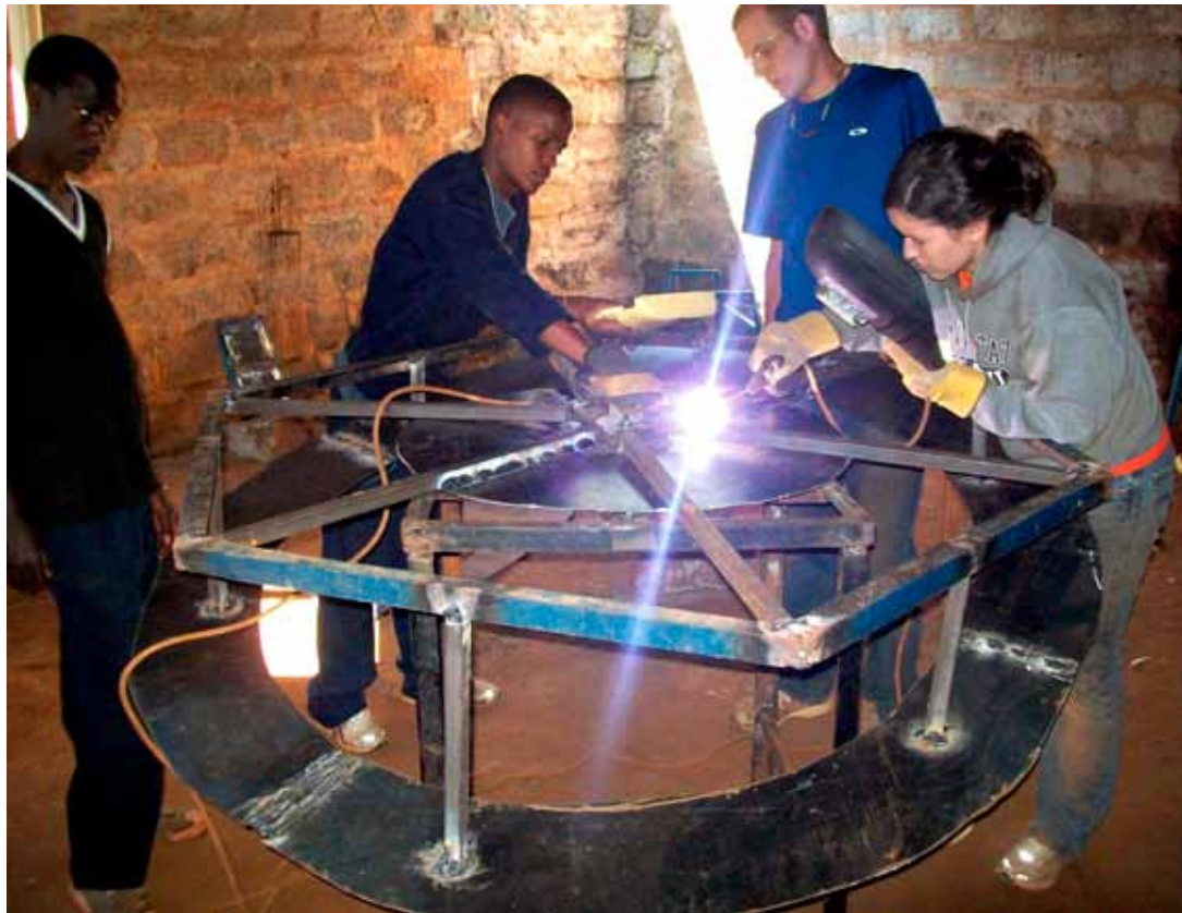
Fabrication of a 'Merry Go Round' water pumping system in Nyeri, Kenya.
